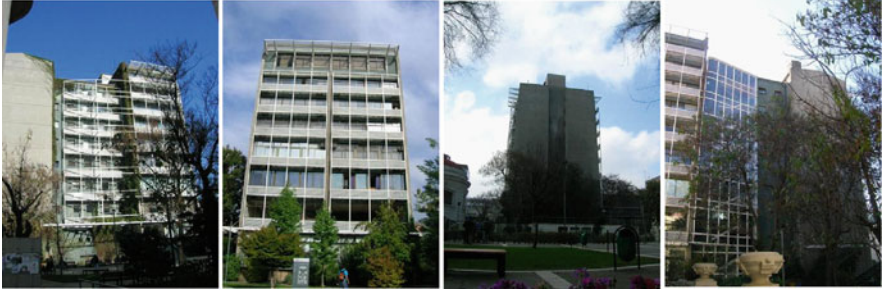
Fig. 8.3 Torre Central general view
