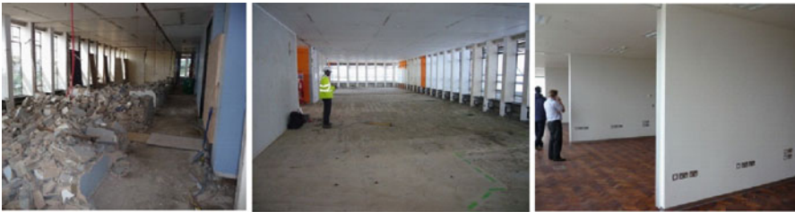
Fig. 6.3 Demolished masonry partitions, cleared floor and new movable partitions
