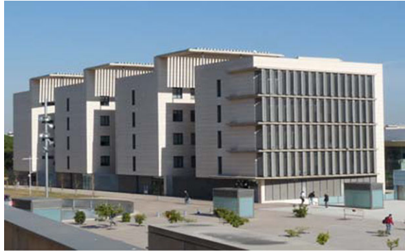
Fig. 17.1 Picture of the block of buildings omega located in the Technical University of Catalonia (BarnaTech) ( above ) and sketch of the 2D structural model ( below )
