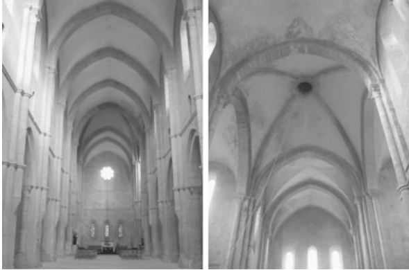
Fig. 21.2 The vaulted system of the Fossanova church
