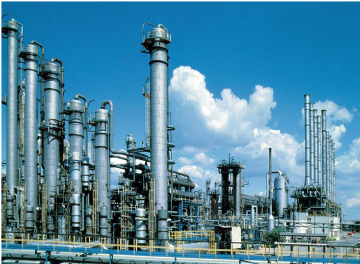
Fig. 2.10 In the aromatics and olefin plant of the Ruhr oil refinery in Gelsenkirchen, e.g. plastic is produced, http://www.deutschebp.de/liveassets/bp_internet/germany/STAGING/home_assets/images/presse/raffinerie_verarbeitung/bild_14690.jpg (retrieved April 8th 2013)
