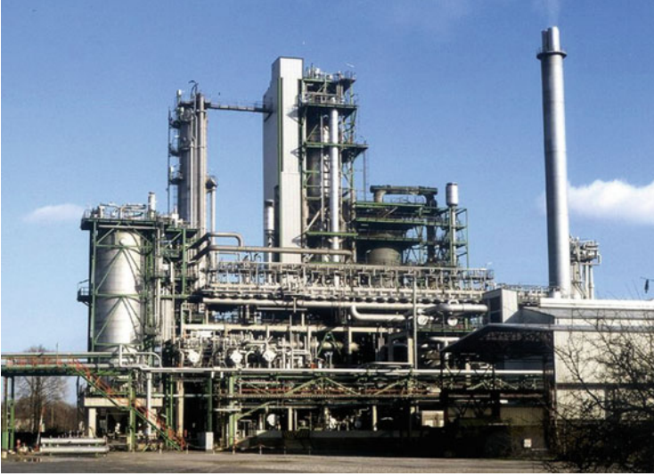
Fig. 2.9 BP operates the second largest refinery system in Germany (Pictured: cracker plant of the Ruhr oil refinery in Gelsenkirchen, http://www.deutschebp.de/liveassets/bp_internet/germany/STAGING/home_assets/images/presse/raffinerie_verarbeitung/bild_14696.jpg ) (retrieved April 8th 2013)
