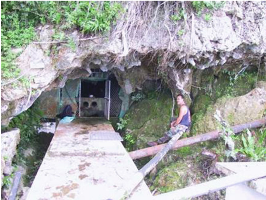
Fig. 13.13 Water cave on Rota provides the primary source for potable water for the entire island. The cave entrance has been modified to impound water and collect it for distribution throughout the island
