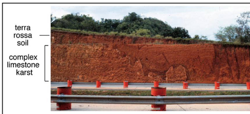
Fig. 6.5 Road cut, northern Puerto Rico, as seen in 1992 when newly made. The overlying grass-covered surface is a uniform slope, but the road cut reveals that the bedrock beneath has a jagged form produced by karstification, with a terra rossa soil overlying it. That soil will compact on the
