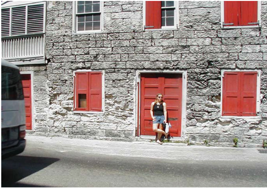
Fig. 8.21 Tafoni present low on the side of a building on a busy street, in Nassau, on New Providence Island. Note the development preferentially close to the ground (Photo by J.E. Mylroie)
