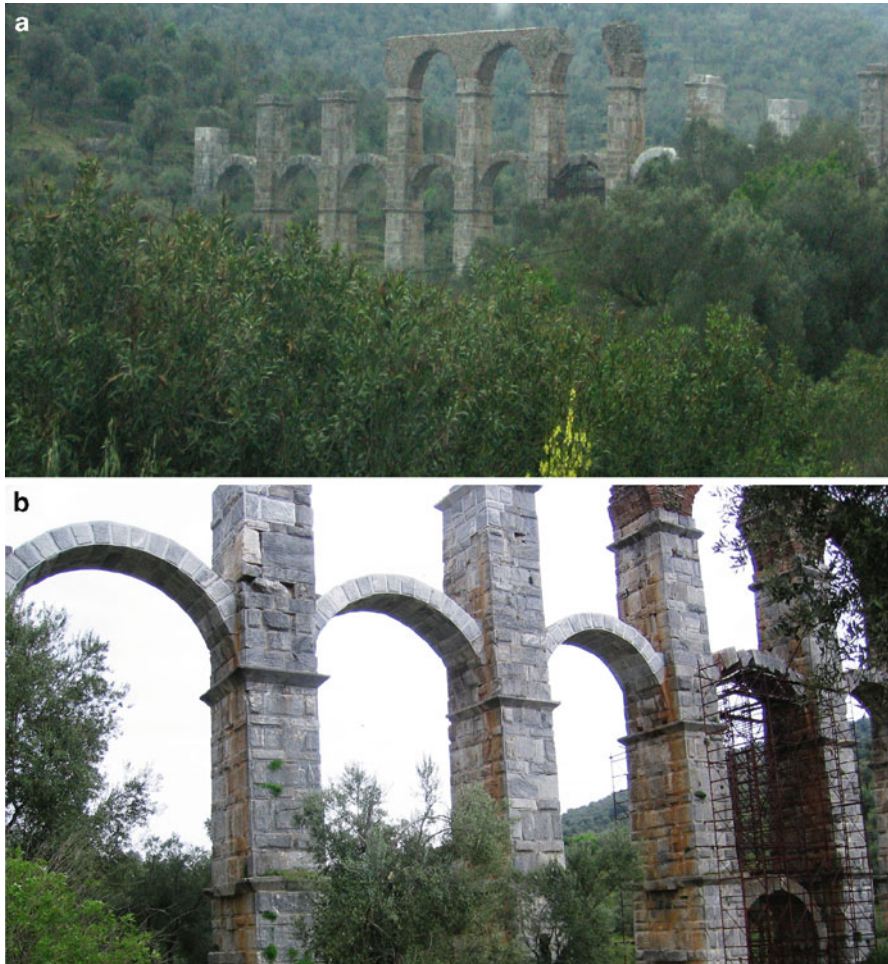
Fig. 2.2 (a) Remains of the Roman aqueduct in Moria, a Lesvian village at 6 km from Mytilene town; (b) Pillars and the arcs of the arches
