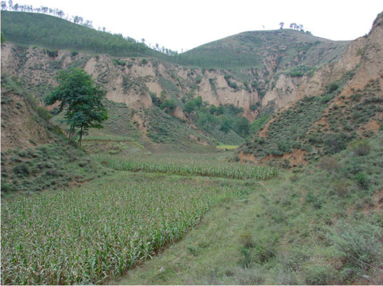
Fig. 5.4 Part of the cascade of check-dam reservoirs in the western main valley in Yangjuangou
