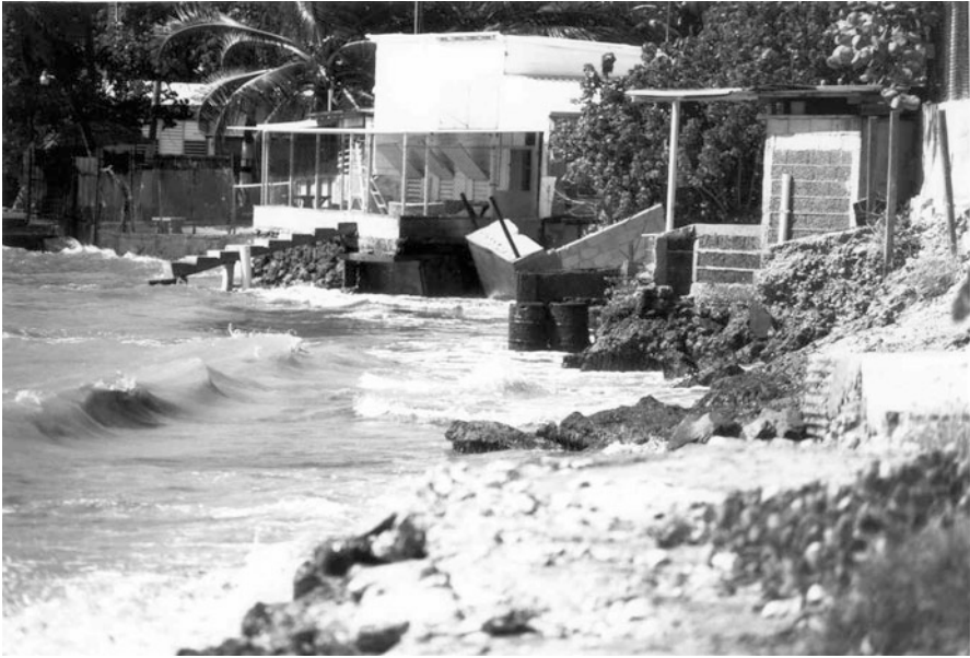
Fig. 4.3 No beach remains in front of these damaged buildings and collapsed portion of small seawalls in front of houses along Route 2 near Balneario El Tuque. The offsets of the closely spaced buildings and hodge-podge structures also have the effect of a groin field (From Bush et al. 2009)
