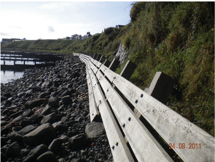
Fig. 6.6 Present (2011) ground view of current (recently upgraded) groynes and palisade barrier in place at Portballintrae's western shoreline, just down-wave from Leslie's Pier
