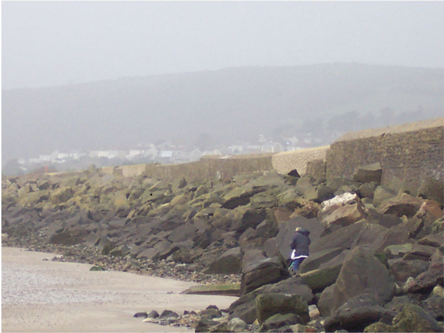
Fig. 17.12 Rock armour protection of rail link
