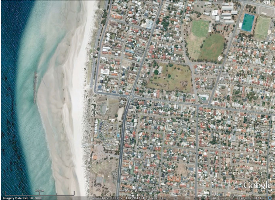
Fig. 2.9 The 200 m long detached Semaphore breakwater constructed in 2005. Note the sand accumulation between the shore and breakwater, and deep rip channel exiting north of the breakwater (Source: GoogleEarth.com)
