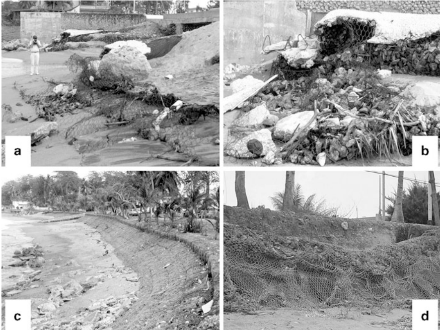
Fig. 4.6 Gabion wall near Aguada's Parque de Colon, built in the late 1980s (From Jackson et al. 2006). (a) and (b) By 1992 the wall had already deteriorated and been "improved" with a concrete covering, which in turn had been broken by storm wave action. Fill rock from the failed gabion was observed to be washed several tens of meters up into the small drainageway visible in upper right of photo a. Sharp, angular cobbles of leaked fill stone and protruding ends of wire strands made the narrowed beach hazardous to walk on. (c) Just to the south, the entire bluff was covered with a sloping gabion revetment/wall, visible in this 1992 photograph. Note that the wire mesh had trapped driftwood and flotsam. The steep wall cuts off the underlying sand scarp sediment source, and increases the erosional effect of waves. (d) By summer of 2000, the gabion in photograph (c) was severely compromised, ruptured and devoid of rock fill over much of its length, and partially slumped and toppled. The scarp was again eroding, providing some new sand to the beach
