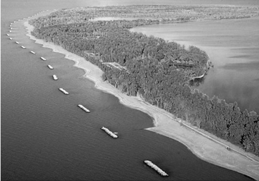
Fig. 9.4 Oblique aerial view of the eastern half of the spit showing the breakwaters and the incipient tombolos extending from the shore. Tombolo formation is quite extensive resulting in an ongoing bulldozing requirement moving around 30,000 cubic yards of sand annually. Photo Courtesy of the US Army corps of Engineers
