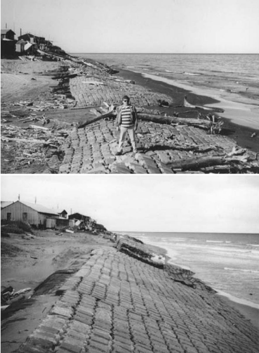
Fig. 5.3 Comparative photographs of 1980s concrete block revetment, upper as failed in 1992, lower , replaced in 1993
