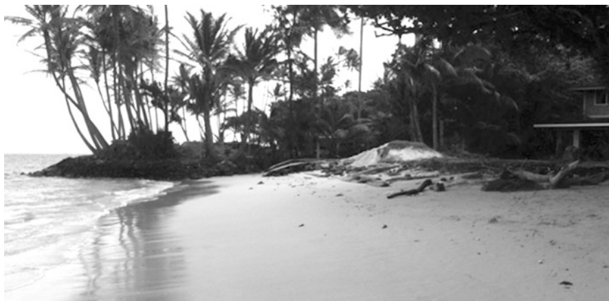
Fig. 10.6 Flanking erosion at Makalii Point (Photo location shown in Fig. 10.5; photo date, March 15, 2011)
