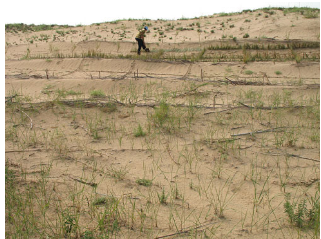
Fig. 12.8 The process of placing the straw checker-board on slopes before inoculation. Qubqi Desert, Dalateqi, Inner Mongolia, August 2008
