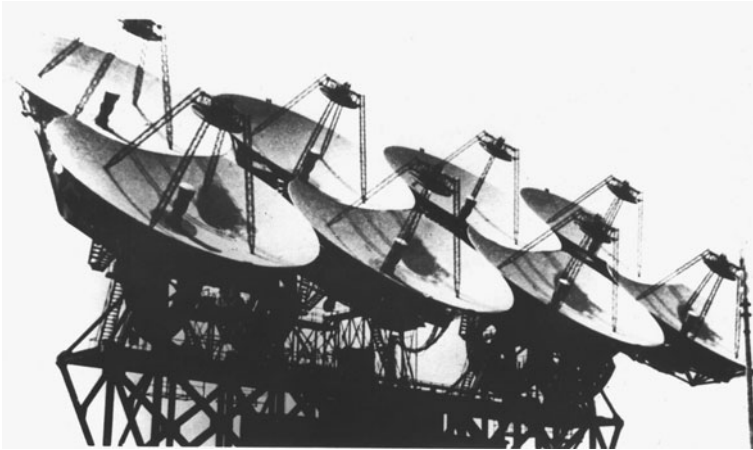
Fig. 9.1 Antenna of the Deep Space Communication Center in the Crimea, consisting of eight parabolic reflectors 16 m in diameter on a common azimuthal–vertical steerable structure
