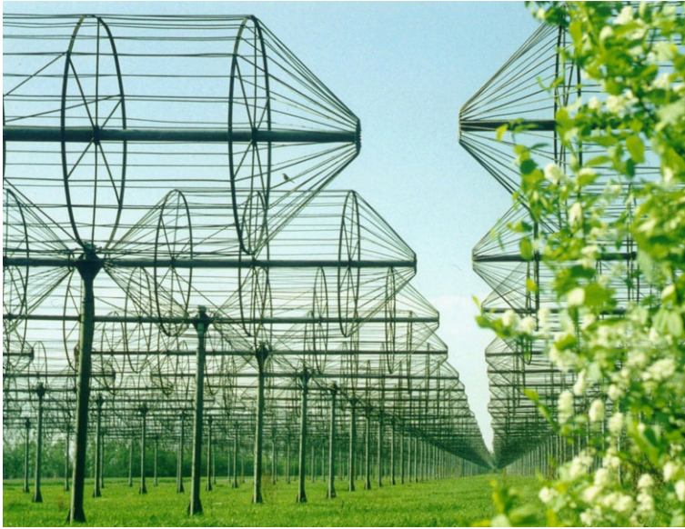
Fig. 8.4 North–South antenna of the UTR-2 radio telescope, comprised of 1440 oscillators
