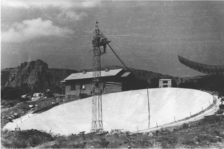
Fig. 1.10 Large fixed centimetre-wavelength radio telescope, with a diameter of 31 m
