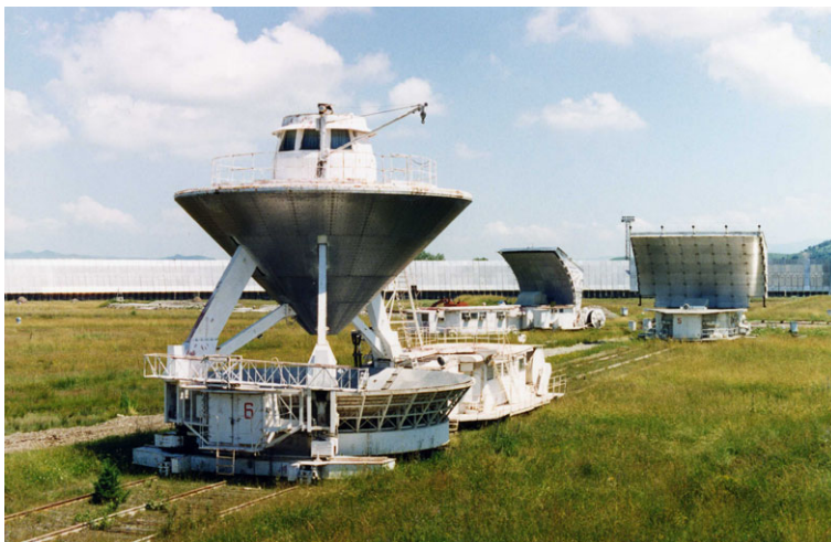
Fig. 5.3 Secondary feed of the RATAN-600 on one of the radial rails
