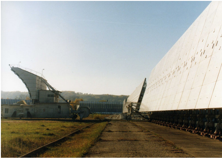
Fig. 5.6 Northern sector of the RATAN-600 circular reflecting surface
