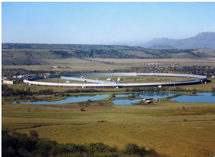
Fig. 5.1 RATAN-600 radio telescope. Circular and flat reflectors, radial rails with feeds and the rotating hub at the centre of the circle, as well as the circular paths in front of the flat reflector. The laboratory building and technical workshop are below and to the left
