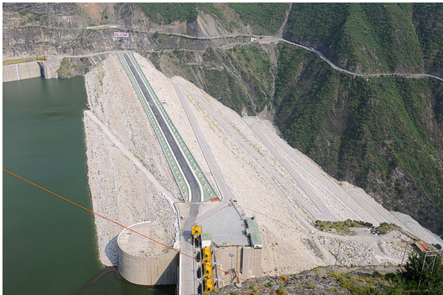
Photo 1.4 Tehri Dam, a rock- and earth-fill embankment dam, at 260 m the highest in India (Photograph: Marcus Nüsser, 15 September 2008)
