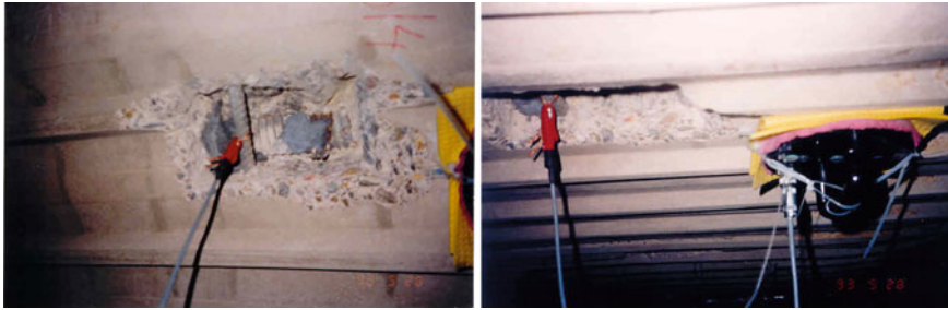
Fig. 7.17 Corrosion rate measured in-situ
