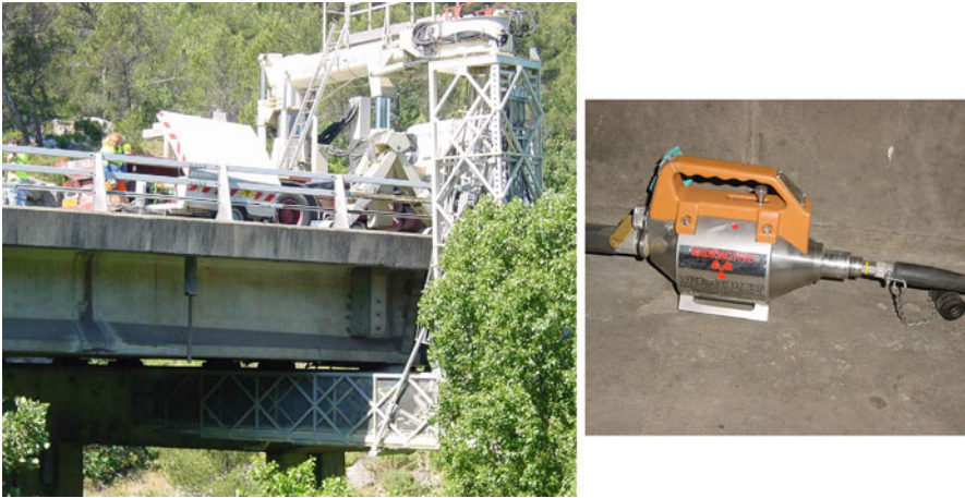
Fig. 7.5 Implementation of the technique at the intrados of a bridge deck (on the left) and a source of Iridium (on the right) – LPC France
