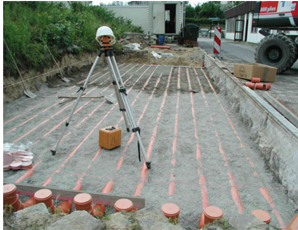
Fig. 6.2 Plastic tubes for Cobalt 60 source at Large Concrete Slab at BAM (after [Taffe et al, 2003])
