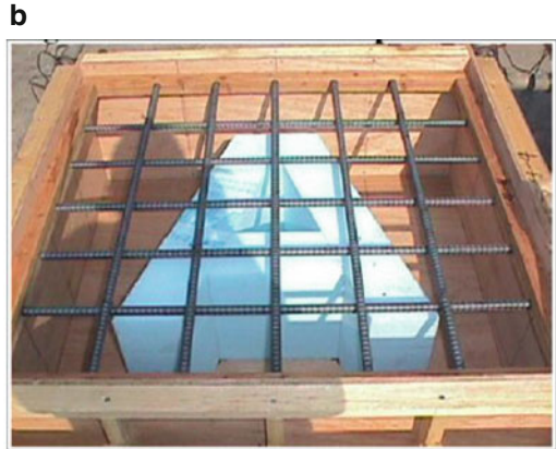
Apperance of specimen before concrete casting
