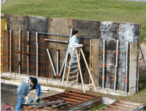
Fig. 4.32 The building of the test wall at LRPC, Lyon
