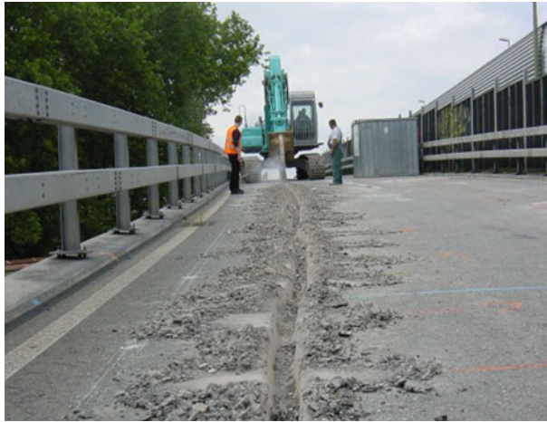
Fig. 4.5 Pavement opening with excavator
