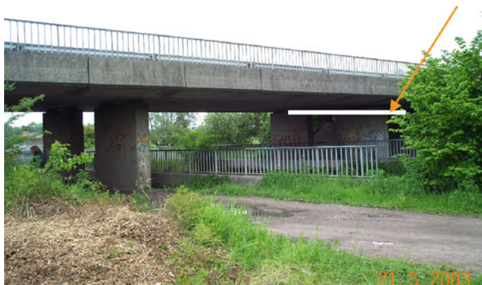
Fig. 1.5 View of the bridge tested with combined techniques. White line below the deck gives location of the profile
