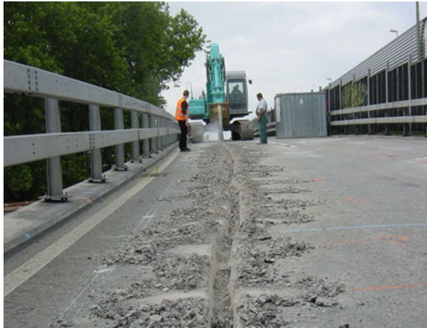
Fig. 4.5 Pavement opening with excavator
