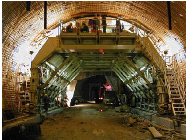
Fig. 4.7 Inner shell of a new tunnel on Germany’s motorway A1
