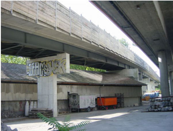
Fig. 4.2 Ramp of Sihl Flyover
