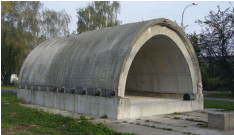
Fig. 4.30 Test tunnel at MFPA Leipzig (after [Taffe and Gehlen, 2007])
