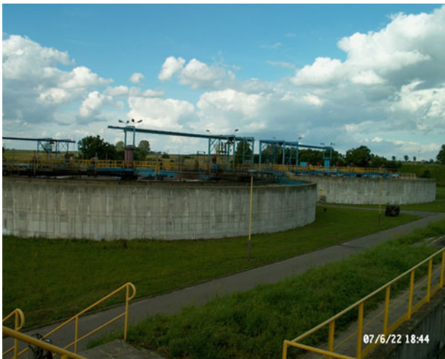
Fig. 3.27 Prestressed concrete storage tanks in Stargard (Poland)
