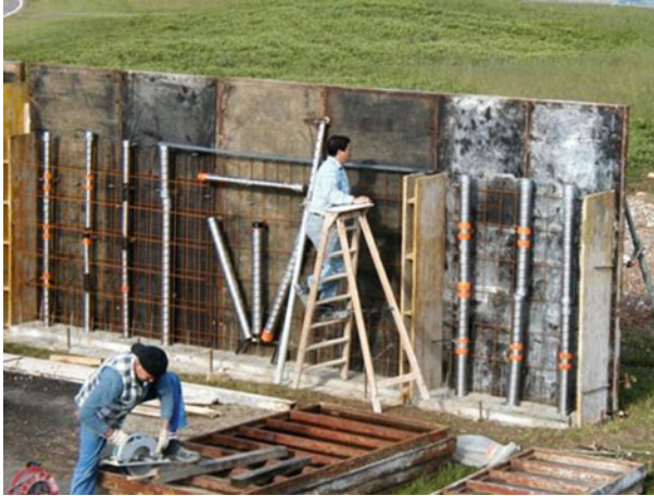
Fig. 4.32 The building of the test wall at LRPC, Lyon
