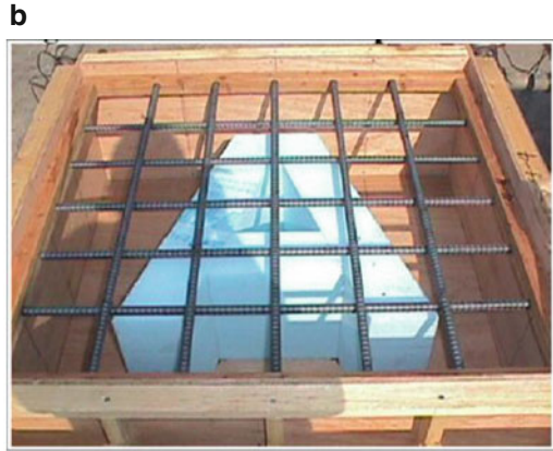
Apperance of specimen before concrete casting
