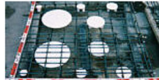
Arrangement of defects
