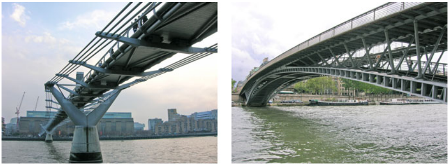
Fig. 1 London Millennium Bridge a and Solferino Bridge in Paris b : two examples of footbridges undergoing the phenomenon of synchronization induced lateral oscillations
