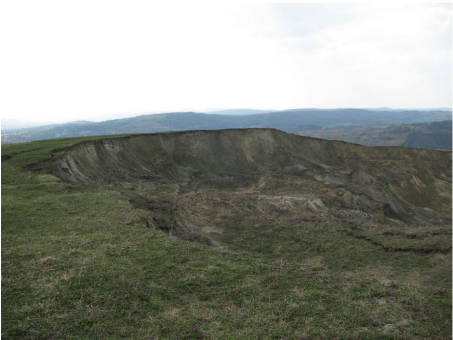
Fig. 10.4 Waste dump affected by a recent deep-seated landslide, Mateești (Getic Subcarpathians) (Photo: Marta Jurcescu)
