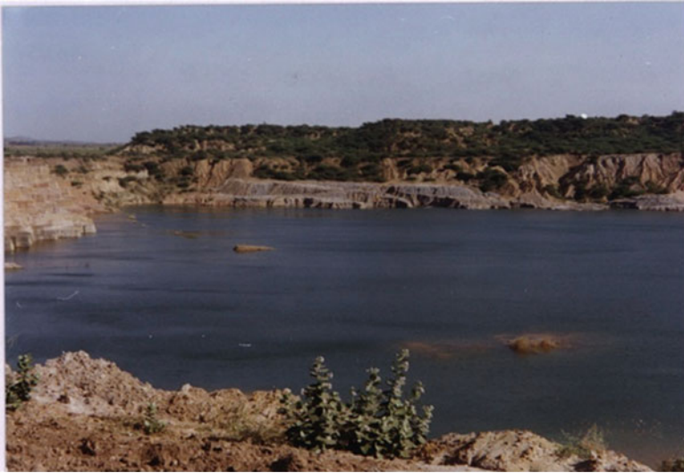
Fig. 32.2 Accumulated acidic water sump at Rajparddi lignite mine
