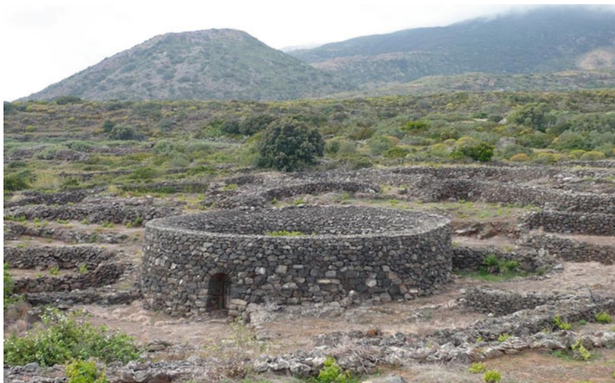
Fig. 13.5 A ‘pantesco garden,’ on the Mediterranean island of Pantelleria (Ben Ryé) between Sicily and Tunisia. The traditional practice of constructing dry-stone walls, which protect trees within them from strong winds, allows the cultivation of trees without irrigation under semiarid conditions (Photo courtesy of Giuseppe Barbera)
