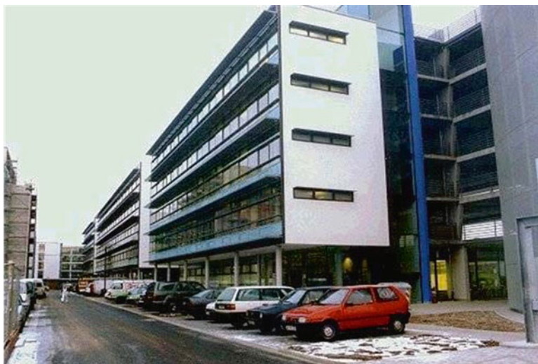
Fig. 7.4 Vilbeler Weg office building, Darmstadt, Germany, 1997/1998 (BIM 2010)
