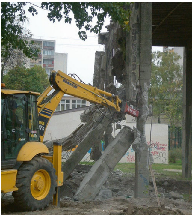
Fig. 7.2 Demolition of a 30 years old concrete structure
