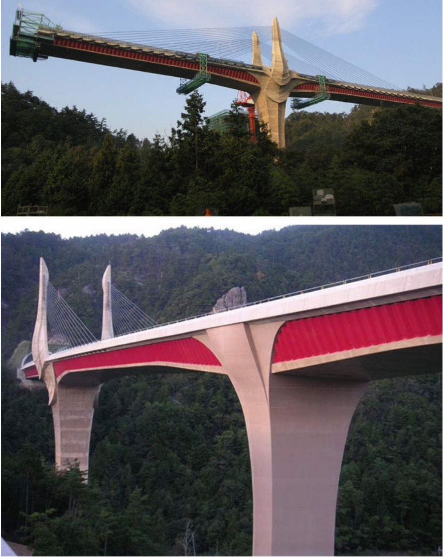
Fig. 22.19 Concrete extradosed bridge with corrugated steel webs
