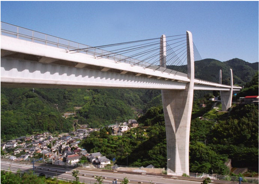
Fig. 21.15 Himi-yume bridge (Courtesy of JH, Sumitomo–Mitsui)
