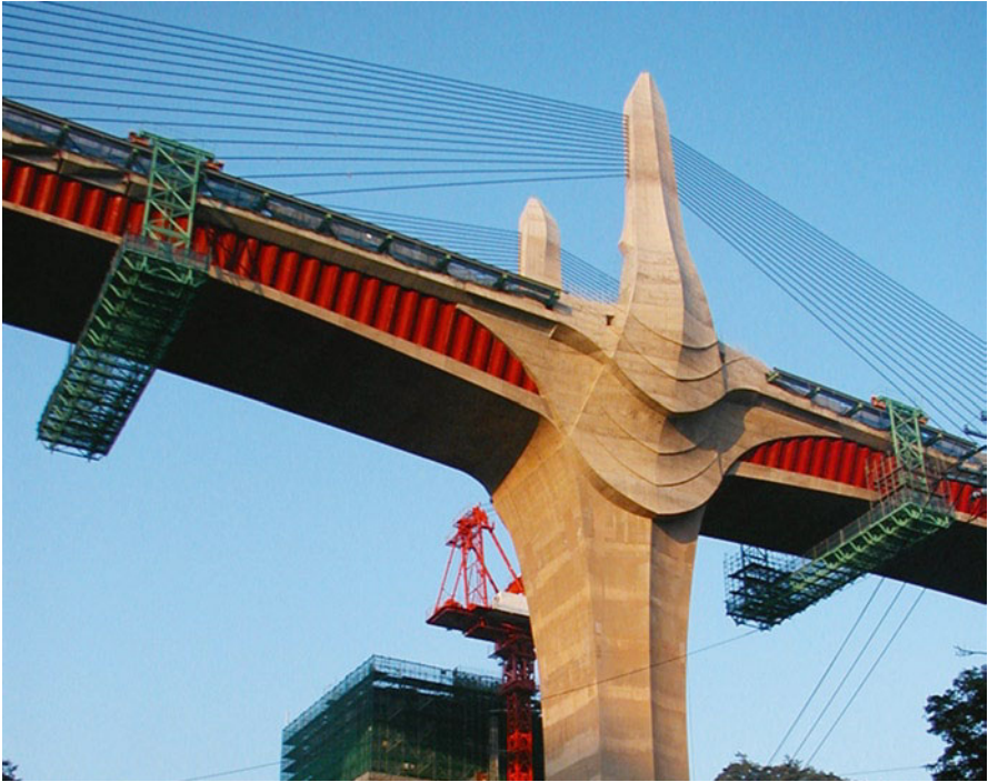
Fig. 21.16 Oumi-ohtori bridge, Frame joint
