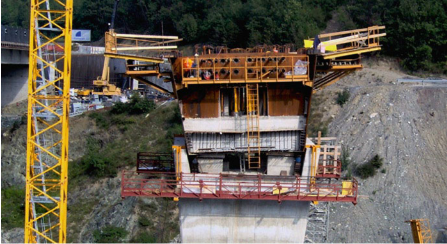
Fig. 23.6 Pier segment assembled on the pier
