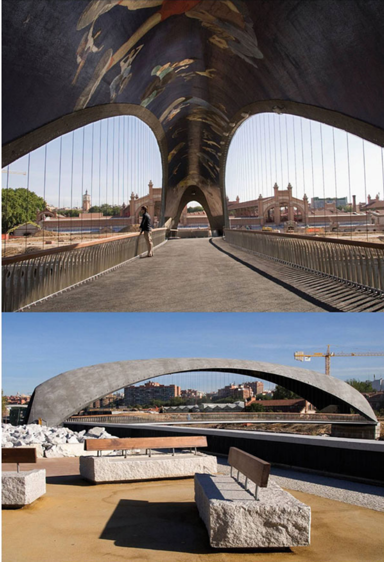
Fig. 2.24 Views of a completed pedestrian bridge
