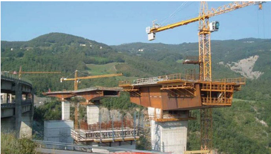
Fig. 23.9 Parallel construction of several hammers
