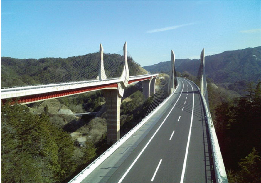
Fig. 21.14 Oumi-ohtori bridge (Courtesy of JH, PS–Mitsubishi)
