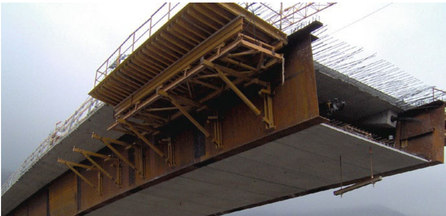
Fig. 23.7 Bottom and top flanges with formwork and scaffolding
