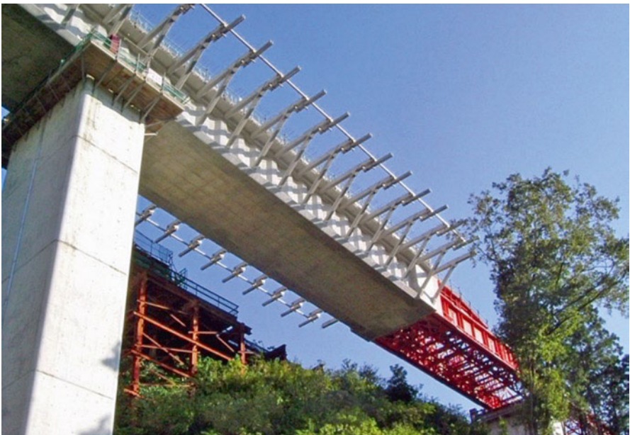
Fig. 21.10 Katsurashima viaduct (Courtesy of JH and Sumitomo-Mitsui)
