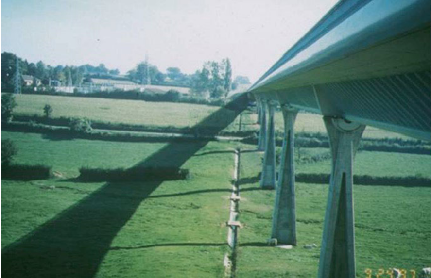
Fig. 21.2 Maupre viaduct near Charolles
