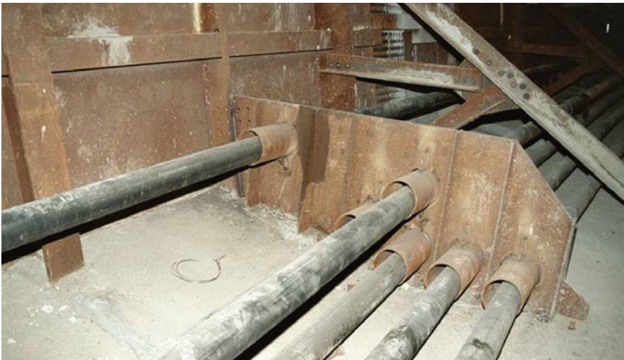
Fig. 23.13 External tendons' deviators
