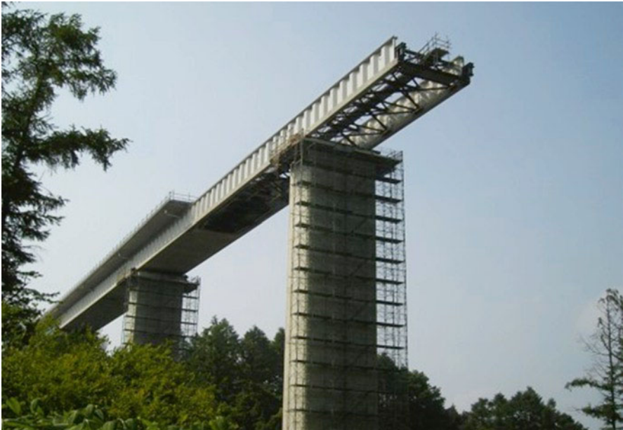
Fig. 21.12 Torisaki-gawa viaduct, launching (Courtesy of JH, Taisei)
