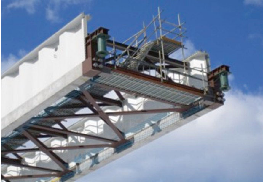
Fig. 21.13 Torisaki-gawa viaduct, launching nose (Courtesy of JH, Taisei)
