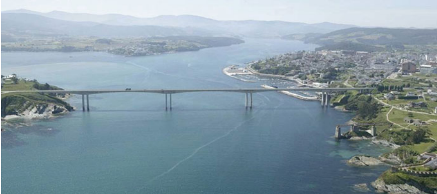
Fig. 2.12 General view of the viaduct before the intervention
