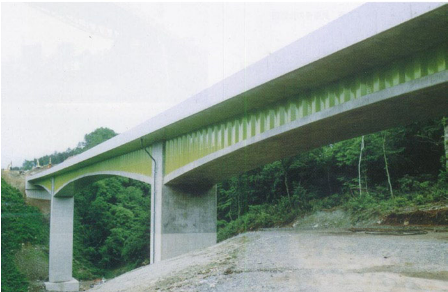
Fig. 22.18 Concrete bridge with corrugated steel web by balanced cantilever segmental construction
