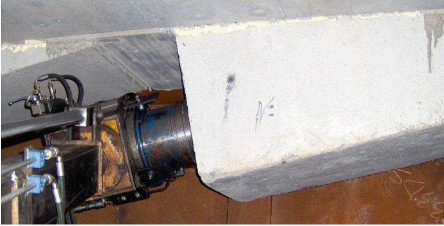
Fig. 23.8 Precast anchorage blisters
