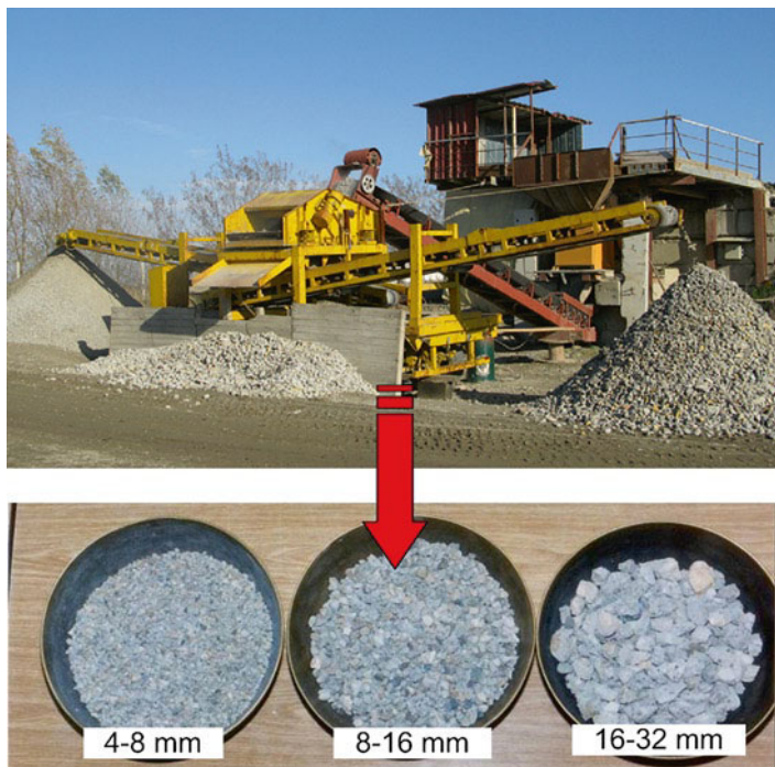
Fig. 7.3 Recycling of demolished concrete in mobile recycling plant
