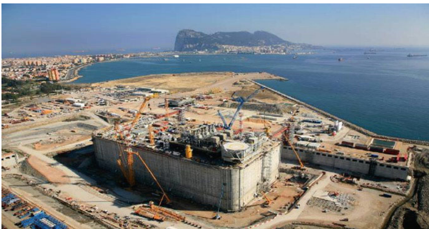
Fig. 20.10 The Adriatic LNG terminal under construction in Spain
