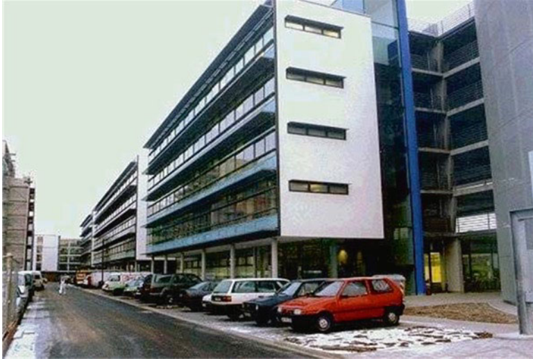
Fig. 7.4 Vilbeler Weg office building, Darmstadt, Germany, 1997/1998 (BIM 2010)
