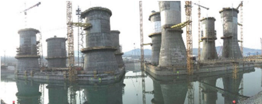
Fig. 20.12 Sakhalin II platforms during construction in Nahodka, Russia
