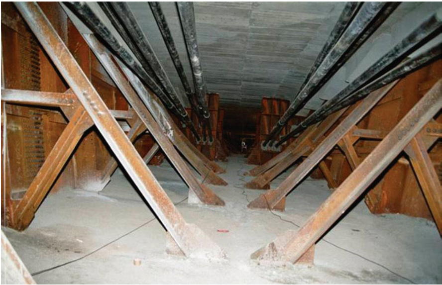
Fig. 23.12 Internal stiffeners
