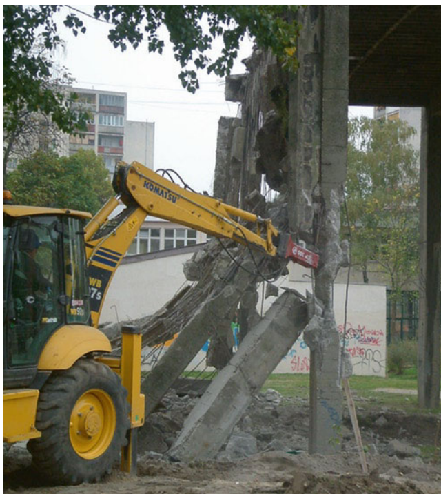
Fig. 7.2 Demolition of a 30 years old concrete structure
