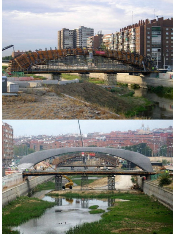
Fig. 2.29 Structure during construction
