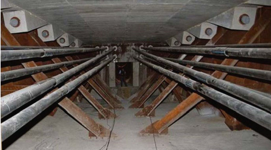
Fig. 23.15 Internal view of external tendons near the pier segment
