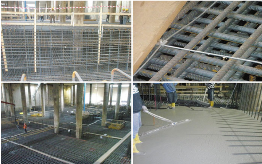
Fig. 2.10 Reinforcement layout and density, and views of casting the self-compacting concrete and of surface finishing
