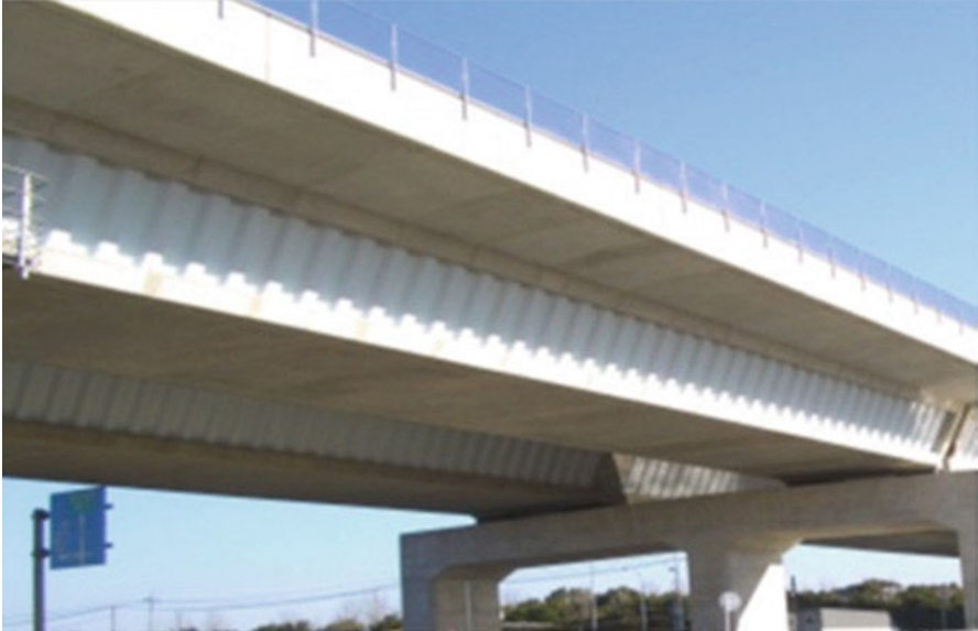
Fig. 22.2 Concrete bridge with corrugated steel webs
