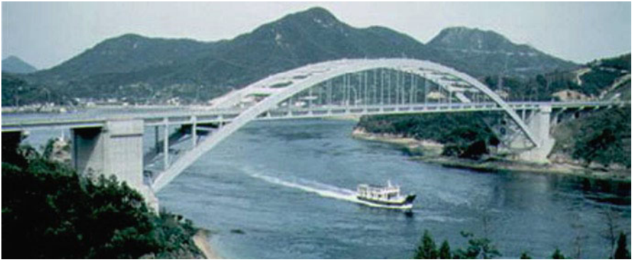
Fig. 22.24 The steel arch bridge (span 297 m) that could be replaced by the extradosed corrugated web bridge
