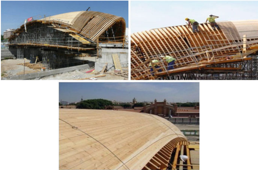
Fig. 2.30 Some details of the formwork
