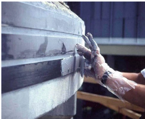
Fig. 9.9 Strengthening of a grain silo with CFRP strips
