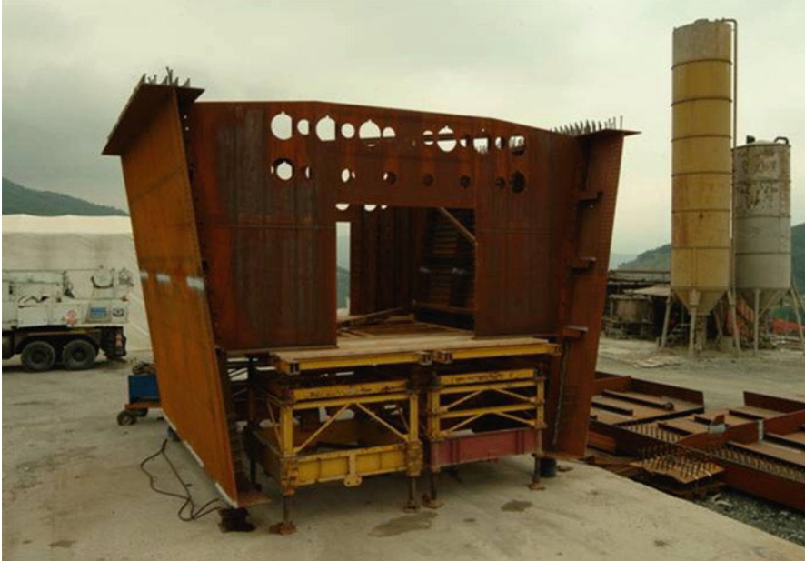
Fig. 23.5 Pier segment ready to be assembled
