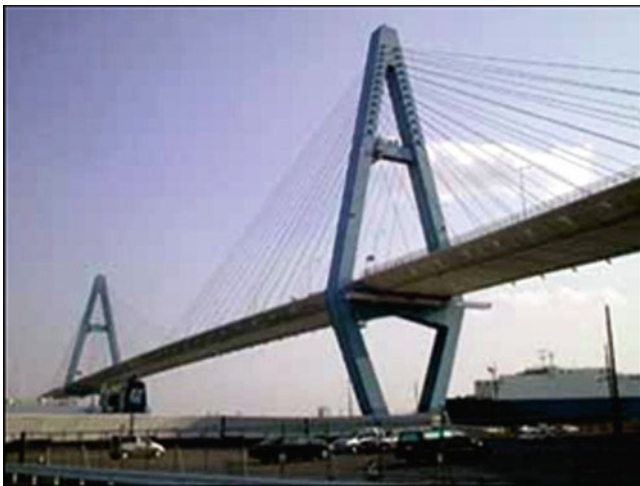
Fig. 22.25 The steel cable-stayed bridge (span 410 m) to be replaced by the extradosed corrugated web bridge
