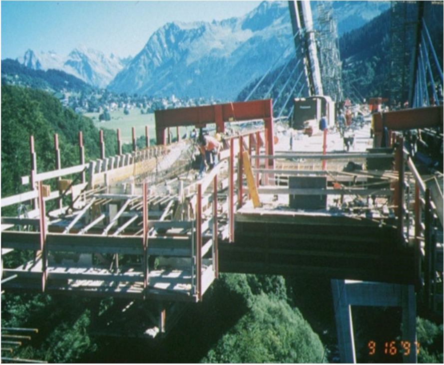
Fig. 21.9 Sunniberg bridge, form traveler
