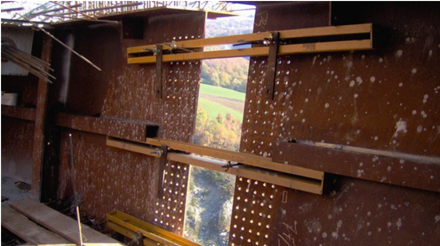
Fig. 23.11 Completed cantilever spanning 60 m
