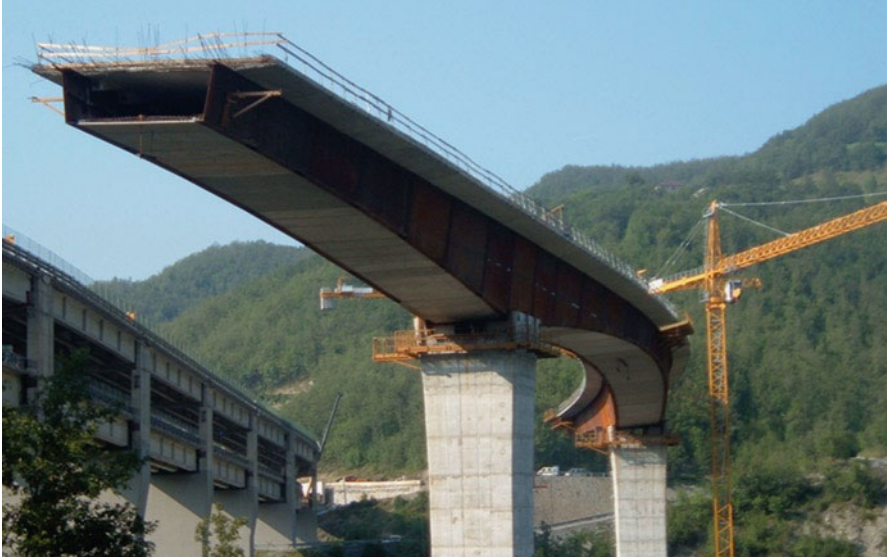
Fig. 23.10 Completed cantilever spanning 60 m
