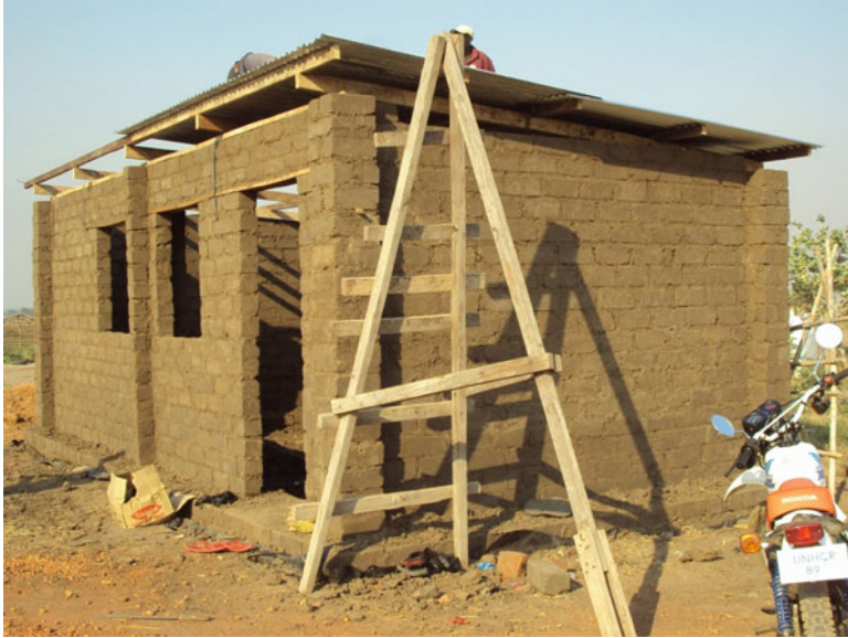
Fig. 8 Stabilized soil block technology in use in Sudan (© Fernando Murillo)
