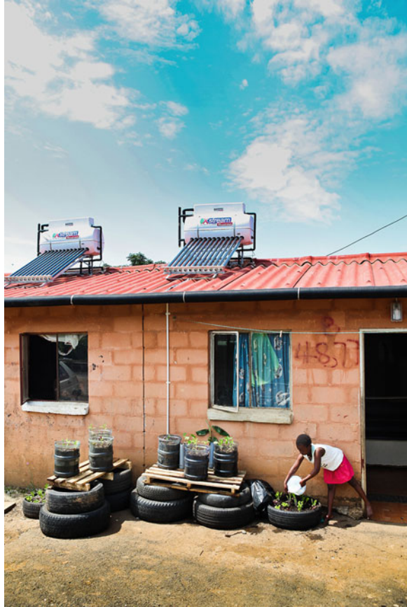
Fig. 6 Retrofitted housing in Cato Manor, Durban, South Africa (© Photo courtesy of Green Building Council of South Africa. Photographer: Willem De Lange)
