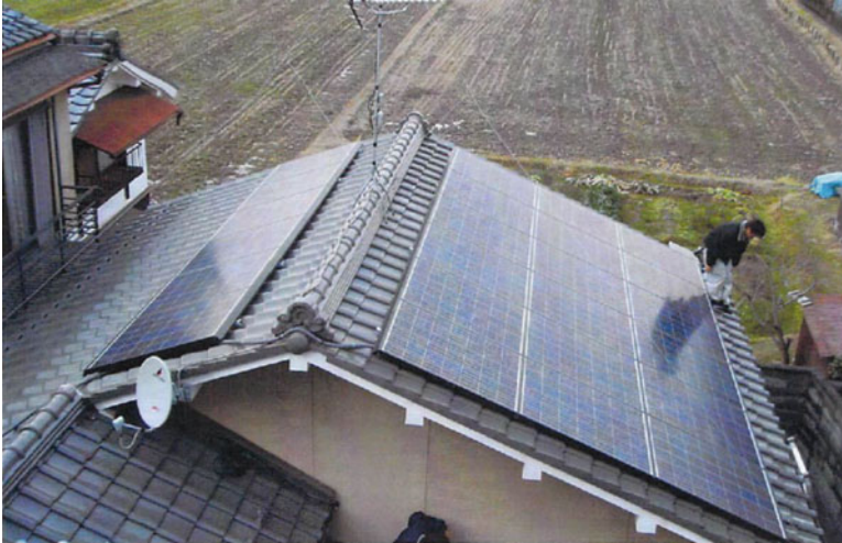
Fig. 4 A photovoltaic panel roof installation
