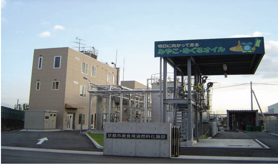
Fig. 8 A Kyoto City facility for used cooking oil fuel established in 2004, producing 5,000 l per day
