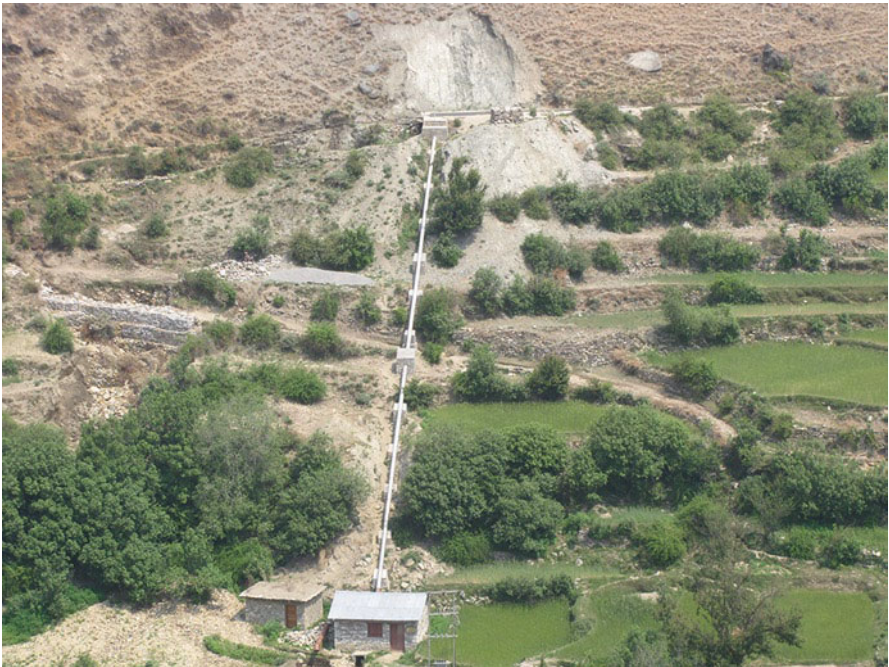
Small hydroelectric power station in the buffer zone of the Shey Phoksundo National Park: involving local people in conservation (Photo by PK Paudel)
