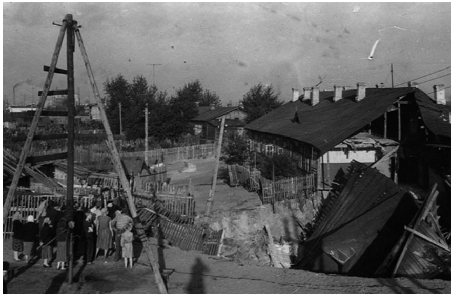
Fig. 4.3 Collapse of a residential building in Nizhny Novgorod region (1959)
