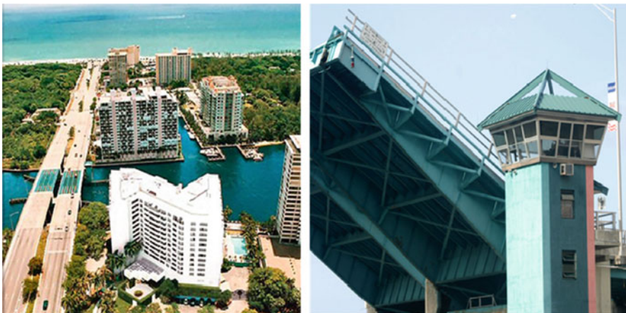
Fig. 2 Sunrise Boulevard Bridge (SBB)
