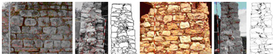
Fig. 6 On site survey of stonework sections
