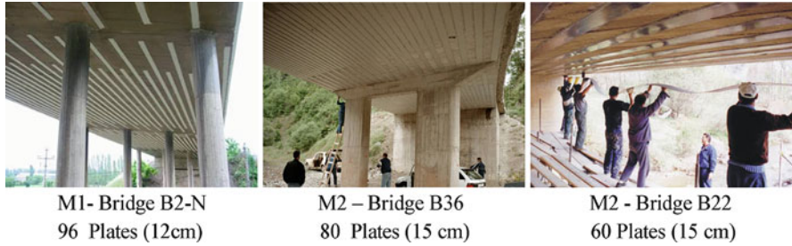
Fig. 1 Typical slab bridges with large CFRP-plate bonded areas
