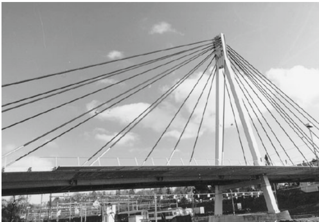
Fig. 13 Cable stayed Stork Bridge in Winterthur crossing 18 tracks of the Swiss Railways
