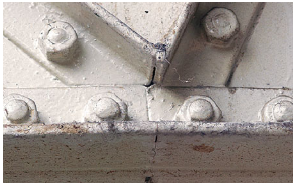
Image 4 Image taken during the tests in the industrial hall. The image, at a height of approximately 20 meter, shows the details of the historic iron construction
