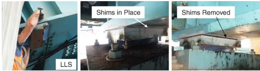
Fig. 4 Live Load Shoe and shim removal
