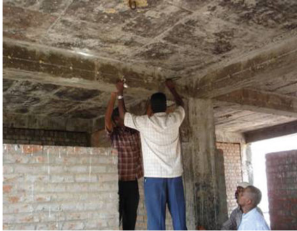
Fig. 1 UPV Test in Progress
