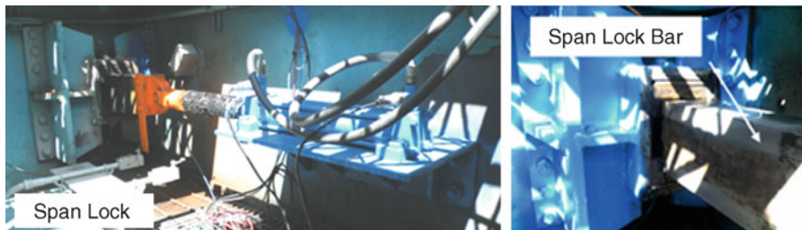
Fig. 5 Span Lock and shim removal
