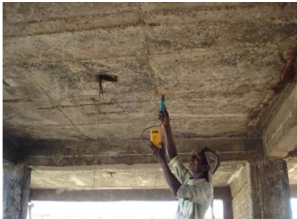
Fig. 2 Half Cell Potential being recorded
