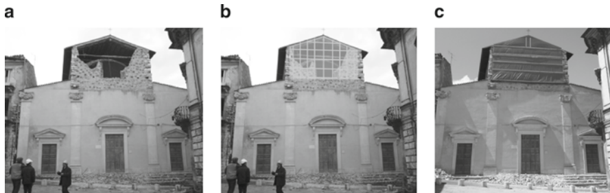
Fig. 2 Collapse of the upper part of the façade (a), design (b) and realization of the intervention (c)
