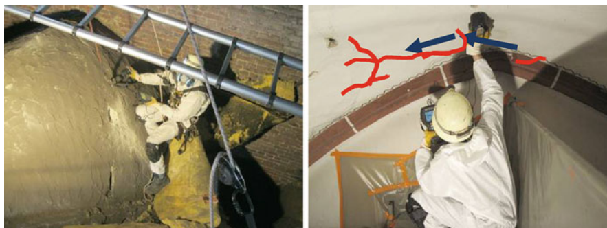
Illustration 4 Left: Measurements on the top of the vault with safety ropes, glass wool was removed; Right: Measurements from the bottom taken while standing on a scaffold
