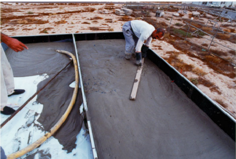
Fig. 2 Installation of roof layers
