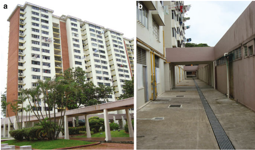
Fig. 8.5 (a) Dawson Estate at Queenstown built in the early 1970s ( top left ); (b) Typical wide space between the slabs in older housing estate ( top right ). Note: The estate is currently too homogeneous and mono-functional; the buildings themselves are not dealing well with the tropical climate, lack proper balconies and western façade shading devices. Today, there are around 900,000 HDB flats across Singapore, housing over 80% of the population (this is around 3.5 million people). HDB has played a unique and significant role over the last four decades and has been crucial to Singapore's urban growth. However, we are now at a point where we have to rethink these existing typical 1960s–1980s new town housing estates, many of which have issues of energy-ineffectiveness and inappropriate, out-dated design lay-outs for living and working in a global city in the tropics
