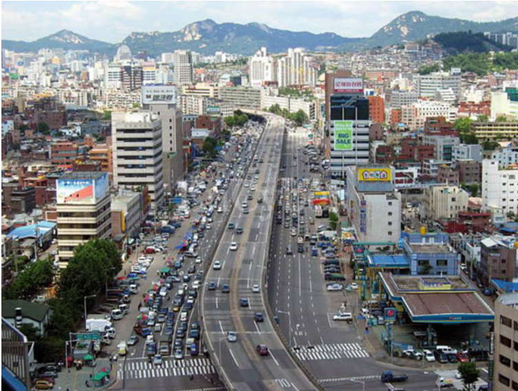
Fig. 5.5 The Cheonggye expressway prior to restoration. Source: The Preservation Institute Web Site www.preservenet.com/.../FreewaysCheonggye.html
