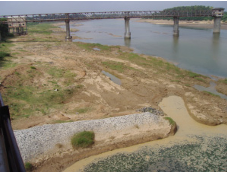
Figure 1.2. A horizontal collector well located within the main course of the Sabarmati River, Ahmedabad, Gujrat, India. (Photo: Courtesy of C. Sandhu, University of Applied Sciences, Dresden)
