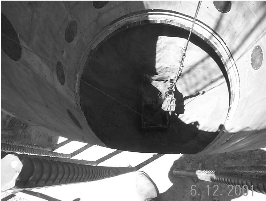
Figure 11.9. Installation of caisson accomplished by removal of material using clamshell excavator.
