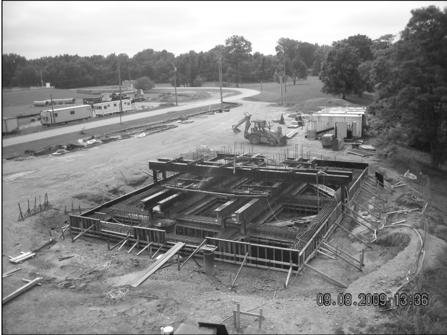
Figure 13.7. Pump station foundation under construction over construction access shaft.
