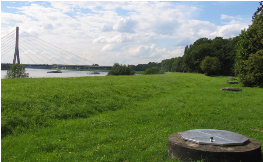
Figure 5.2. Vertical wells at Flehe waterworks and the River Rhine.
