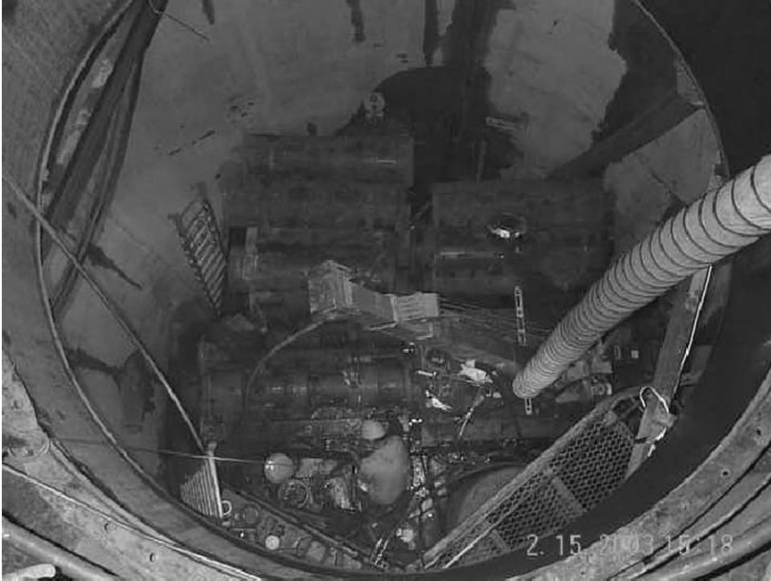
Figure 11.14. Drilling operations during LLDL installation.
