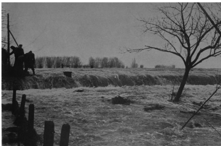
Fig. 83.7 Impact of the 1953-flooding disaster in Zeeland causing about 400 km (250 mi) of dike to breach and flooding at least 1,920 km 2 (475,000 acres)
