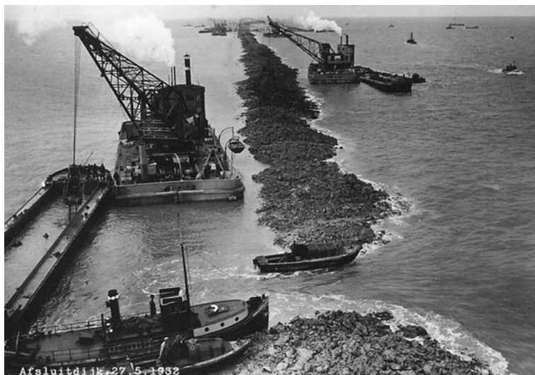
Fig. 83.5 The final stage of completing the Closure Dike (Afsluitdijk) in 1932
