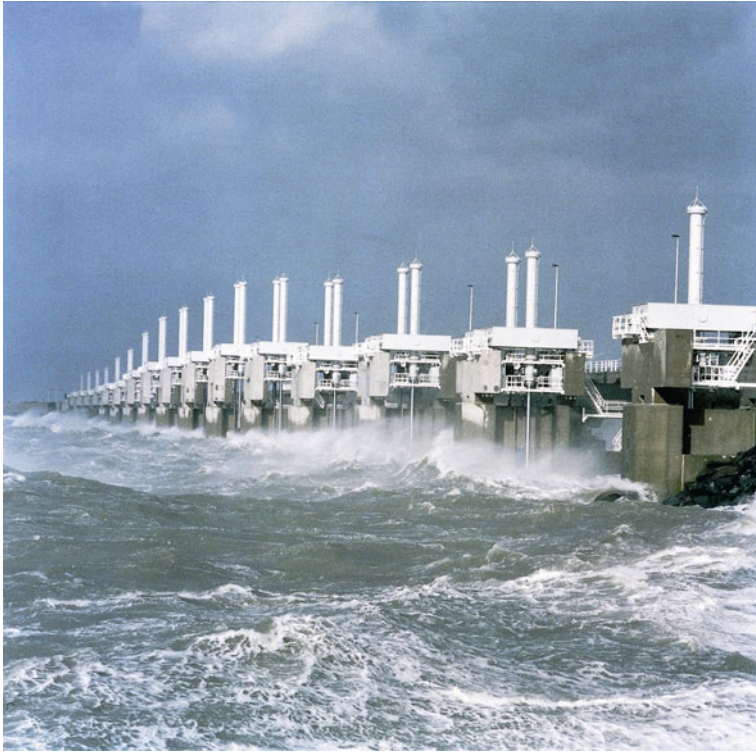
Fig. 83.9 Delta Works: The Storm Surge Barrier is built with a number of large slides held in between piers which can be moved. Normally, the slides are lifted in order to reduce the tides' impacts, except for extra high tides or during severe storm surges when the slides can be entirely lowered (Courtesy Rijkswaterstaat)
