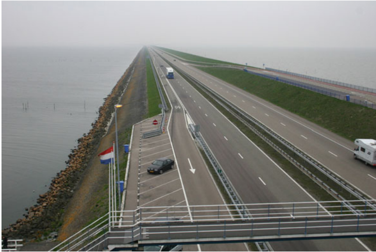
Fig. 83.6 The 32 km (20 mi) long Closure Dike has not really changed shape since the completion in 1932, in spite of modern busy traffic as this photograph from 2006 shows
