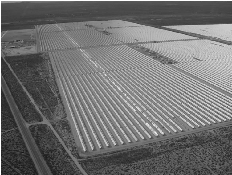
Fig. 27.10 SEGS (Solar Energy Generating Plant) at Kramer junction, west of Barstow, California. These installations are concentrating solar power facilities, using parabolic trough with single-axis tracking. They occupy a low-priority patch of land. Source: Wikipedia Commons. http://upload.wikimedia.org/wikipedia/commons/4/44/Solarplant-050406-04.jpg
