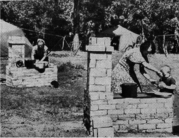
Fig. 15.4 Constructing outdoor stoves in the virgin lands. (Source: Brezhnev, 1978)
