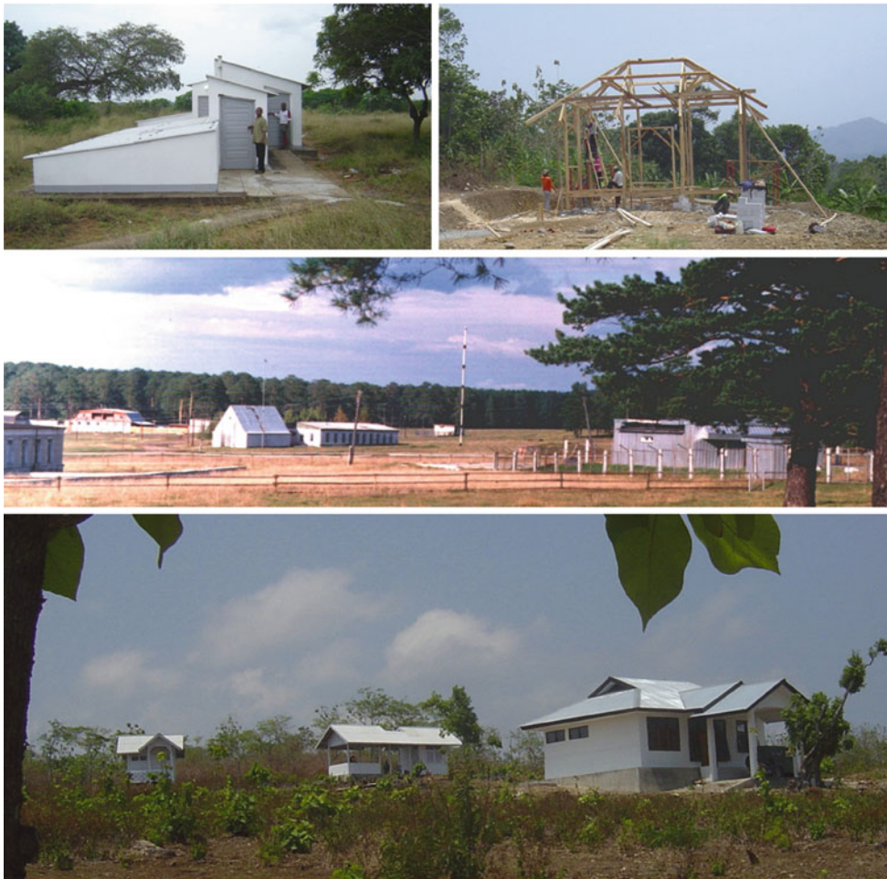
Fig. 1.2 Pictures of INDIGO installations. Top: Variometer house at Maputo, Moçambique. The newly erected variometer house in Pelabuhan Ratu, Indonesia. Middle: Arti observatory in Russia. Bottom: the new Kupang observatory in Timor-West, Indonesia
