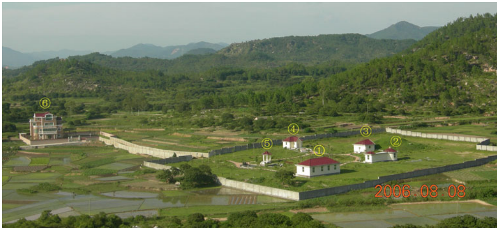
Fig. 1.6 Overview of the Quanzhou magnetic observatory. 1: Absolute house, 2: Proton vector magnetometer hut, 3: Variation room, 4: Electric hut, 5: Instrument comparison hut and 6: Office
