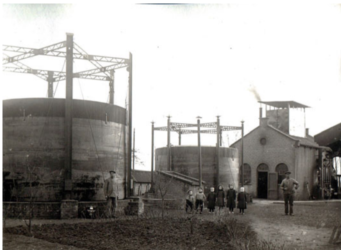
Fig. 1.1 The former gas works 'Delfse Wallen' in Zoetermeer, the Netherlands, around 1908, as an example of an activity that often caused contamination of soil and groundwater (photo: Historical Society 'Oud Soetermeer'; reproduced with permission)
