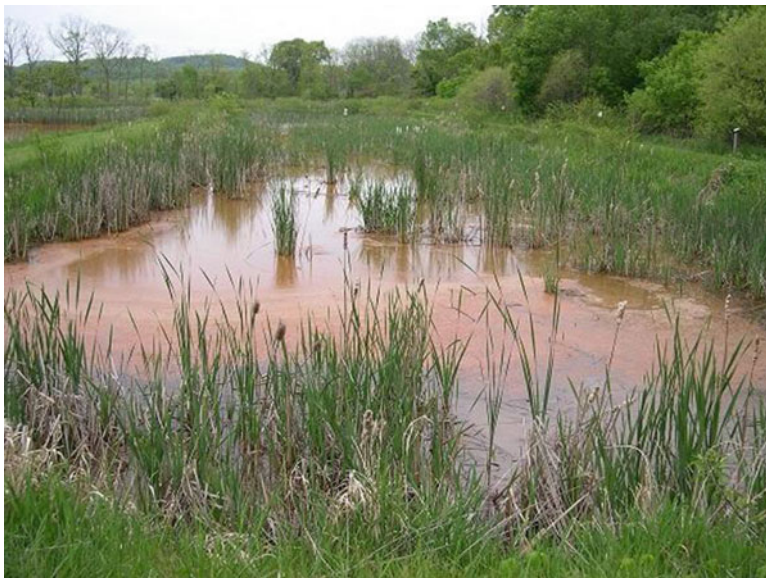
Fig. 2 FWS constructed wetlands for treatment of coal mine drainage at Monastery Run, Pennsylvania, USA, planted with Typha latifolia (Photo credit: Jan Vymazal © copyright remains with the author)
