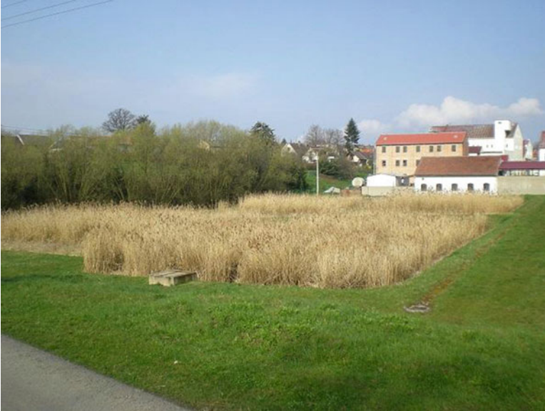
Fig. 4 Constructed wetland with horizontal subsurface flow for 800 PE (population equivalent) at Čistá, Czech Republic planted with Phragmites australis (Photo credit: Jan Vymazal © copyright remains with the author)
