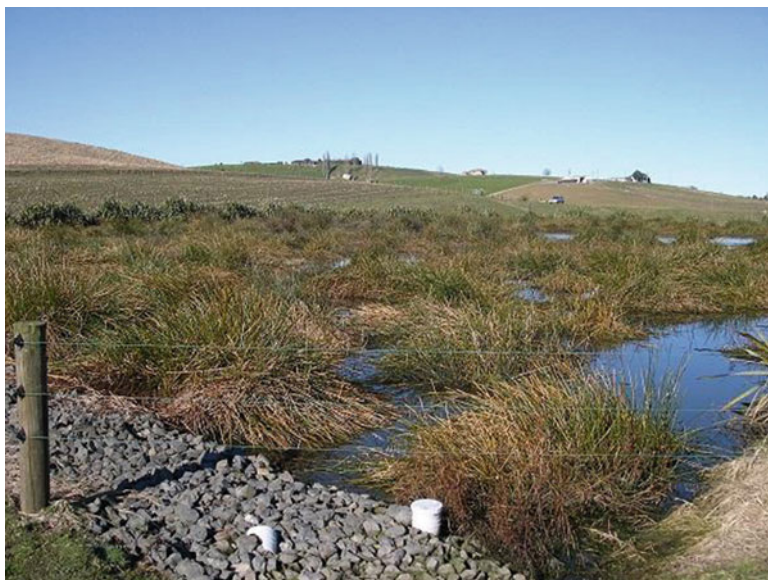
Fig. 1 FWS constructed wetland at Otorohanga, New Zealand, planted with Eleocharis sphacelata for tertiary treatment of municipal sewage (Photo credit: Jan Vymazal © copyright remains with the author)
