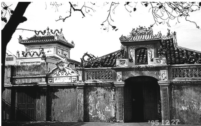
Photo 6.2 Main buildings before restoration at Van Thuy Tu, Phan Thiet City, Binh Thuan Province, Vietnam
