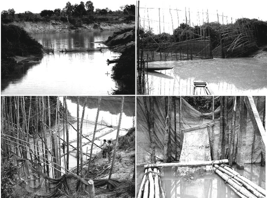
Photo 5.2 Details of barrage construction
