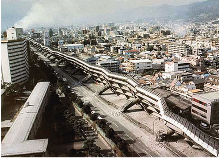
Fig. 10.9 Collapse of the Hnshin Expressway, Kobe earthquake, 1995
