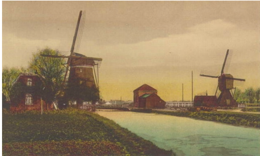
Fig. 17.4 An octagonal mill (left) and a post mill, with a modern pumping station in between
