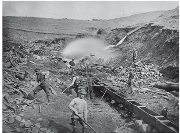
Fig. 24.3 Late nineteenth-century view of placer mining in Illinois Gulch. Water is piped to the site and mixed with sediment along the length of the wooden rocker box in the center foreground to separate out placer metals. (Photograph courtesy of the Colorado Historical Society)
