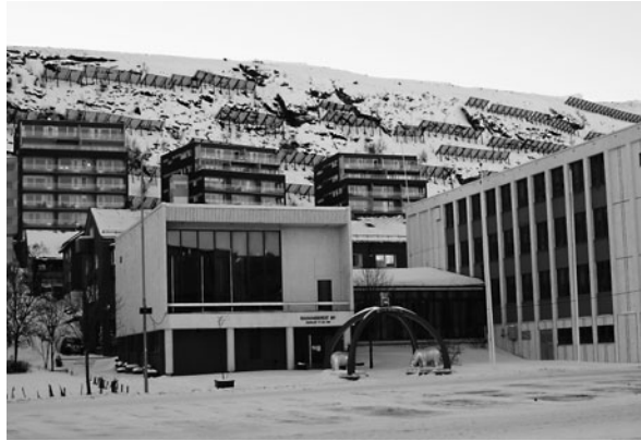
Fig. 2.7 Avalanche protection in Hammerfest. (Photo: Grete K. Hovelsrud)
