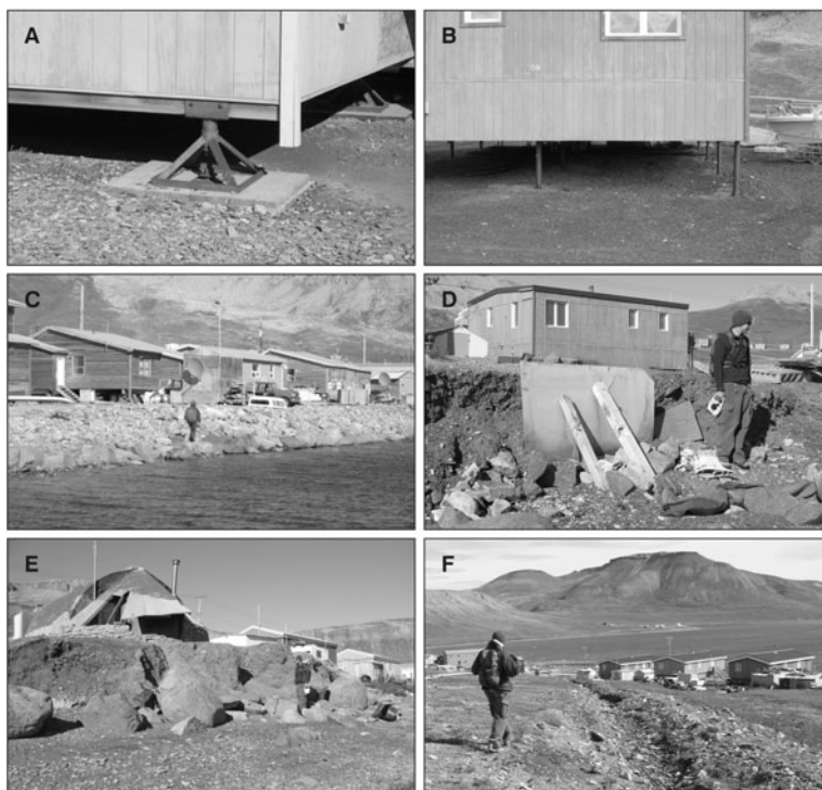
Fig. 5.3 Examples of local adaptation to landscape hazards in Arctic Bay. Adjustable jack (a) and pile (b) foundations mitigate the impacts of permafrost thaw and ground subsidence or heaving on buildings. Coastal armouring, either through large government-funded stabilization projects (c) or local protective measures (d, e), attempts to reduce the impact of erosion on infrastructure and land use. In the cases of (d) and (e), measures were only temporary and erosion eventually undermined local infrastructure. Surface drainage is contained and routed through the community using open ditches (f) and culverts. Photos: Trevor Bell
