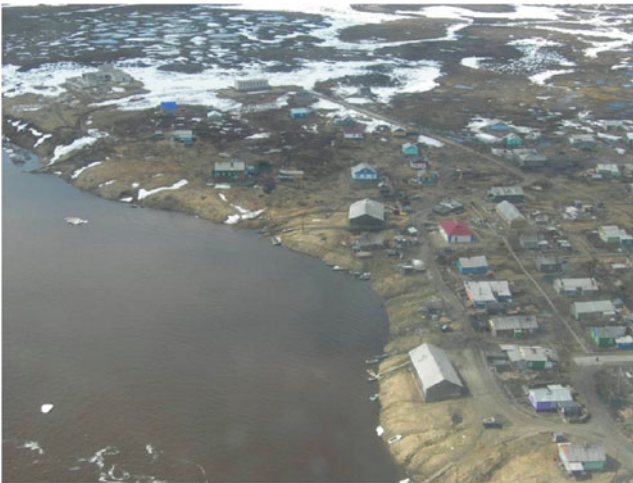
Fig. 6.2 Nelmin Nos on the Riverbank erosion poses an immediate threat for any structures built too close to the river. A few houses, which previously stood on the riverbank, have already been moved and a part of the graveyard has been washed out. The Pechora River is also the only ground transport line that allows passage between the village and the outside 'world', and melt-freeze cycles crucially influence local inhabitants' livelihoods. Photo: Anna Stammler-Gossmann
