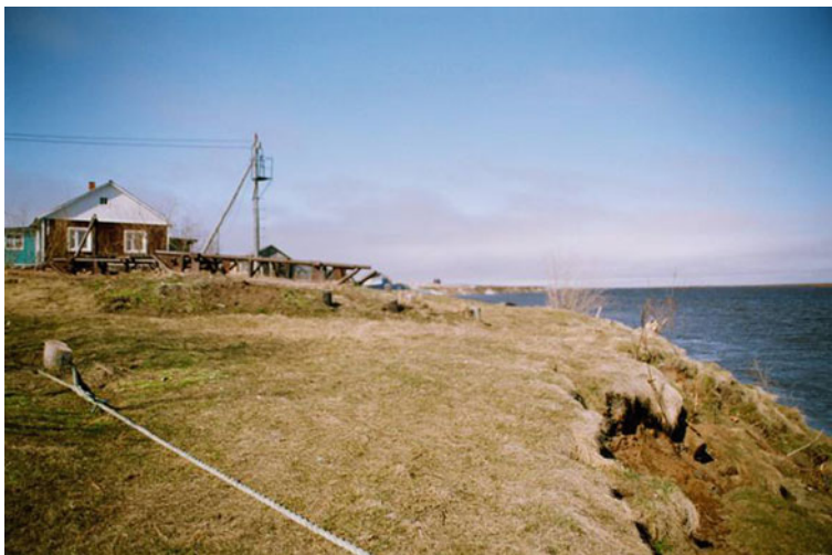
Fig. 6.8 Pechora River Bank erosion in 2008: Removed house (Photo: A. Stammler-Gossmann)
