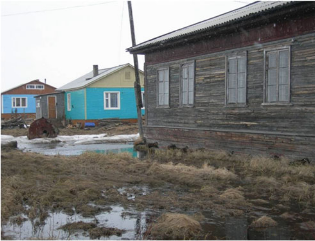
Fig. 6.1 Nelmin Nos. Ever-moving landscape. Swampy tundra terrain presents substantial challenges to the preservation and development of infrastructure in the village. The transition from nomadic to sedentary mode of life in Malozemelskaia tundra, forced by the Soviet state, did not consider adapting housing standards to the tundra landscape. Many houses suffer from damp and shifting foundations. For Nenets reindeer herders, who move between the village and tundra camp, the village still perpetuates an image of a temporary arrangement thus house maintenance has a low priority amongst other activities. Photo: Anna Stammler-Gossmann
