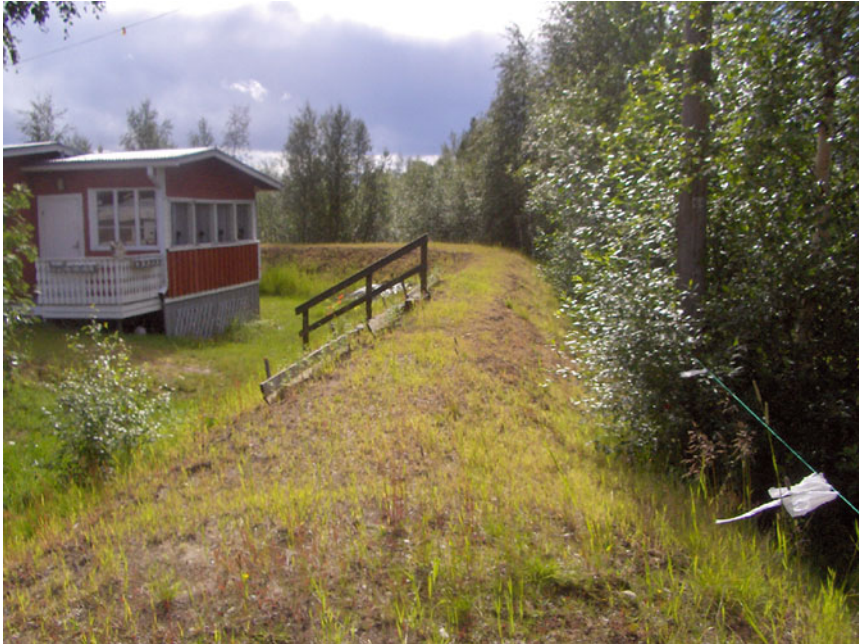
Fig. 9.1 The flood banks are built close to houses in Ivalo. Photo: Reija Valle
