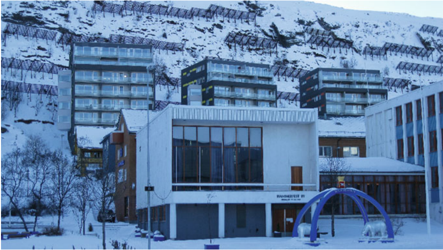
Fig. 2.7 Avalanche protection for apartment buildings nestled against the steep hills in downtown Hammerfest, Finnmark, Northern Norway. Photo: Grete K. Hovelsrud/CICERO
