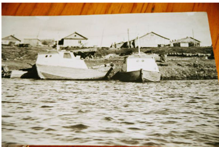
Fig. 6.7 Pechora river bank in 1970s (Photo: A. Stammer-Gossmann, Nelmin Nos archive)
