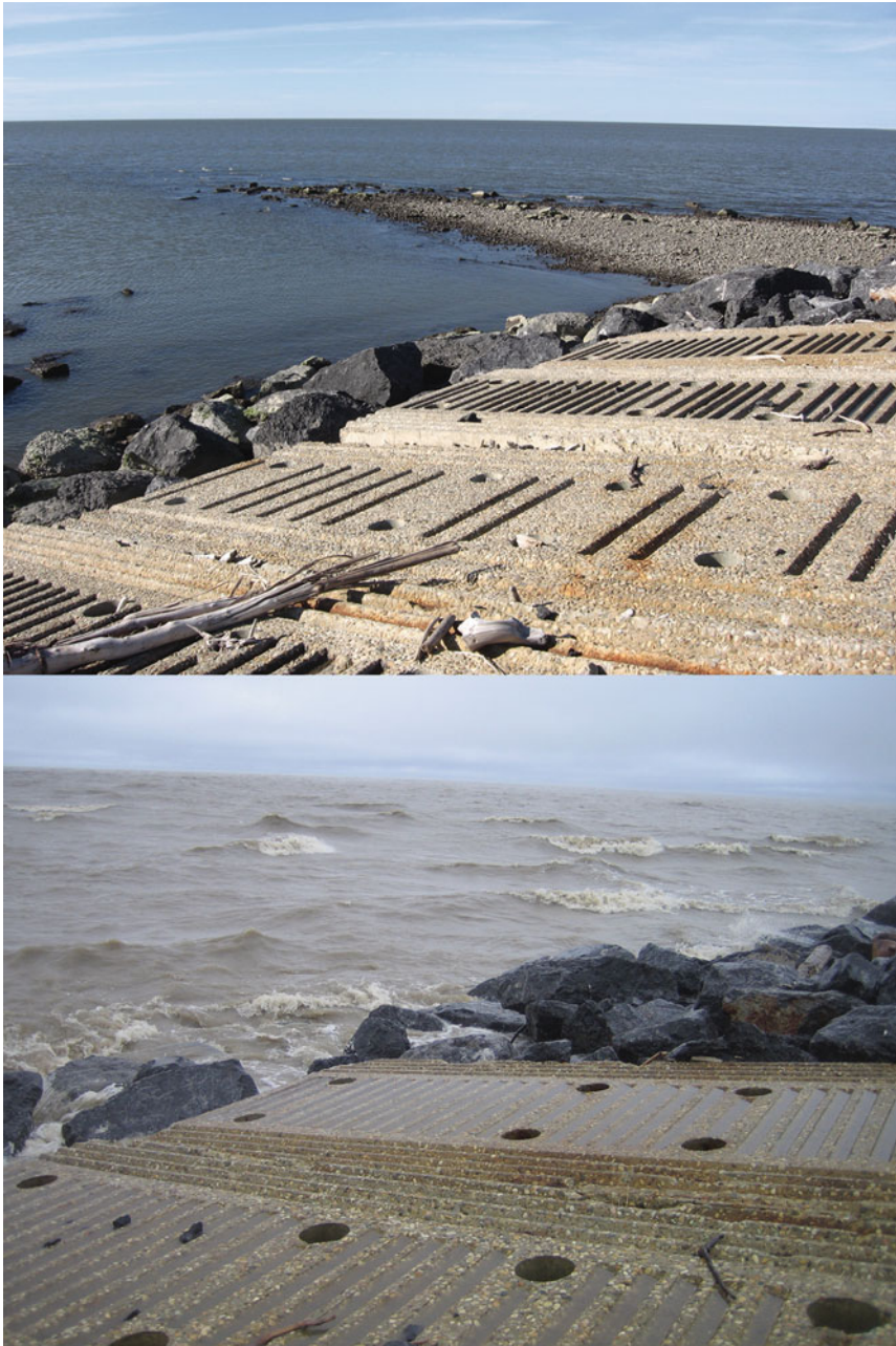
Fig. 3.4 The community of Tuktoyaktuk has used large concrete slabs and boulders to protect the shoreline and slow erosion. The top photo shows the water level on a calm day, exposing the loose small gravel that makes up the original shoreline and underlies the entire community. The bottom photos shows the water level and waves during a moderately strong wind storm in summer 2007. Photo: Mark Andrachuk
