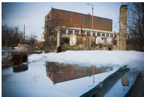
Fig. 1. The machine room of heliostation, built in 1985.
