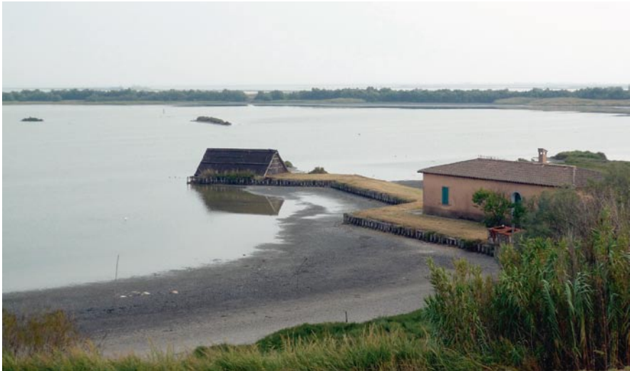
Fig. 1.3 Remaining coastal lagoon Valle di Comacchio (Ferrara, north-eastern Italy): a wood and reed house once used by fishermen and a “casone” (big brick house) used for aquaculture activities (Photo by Scapini)
