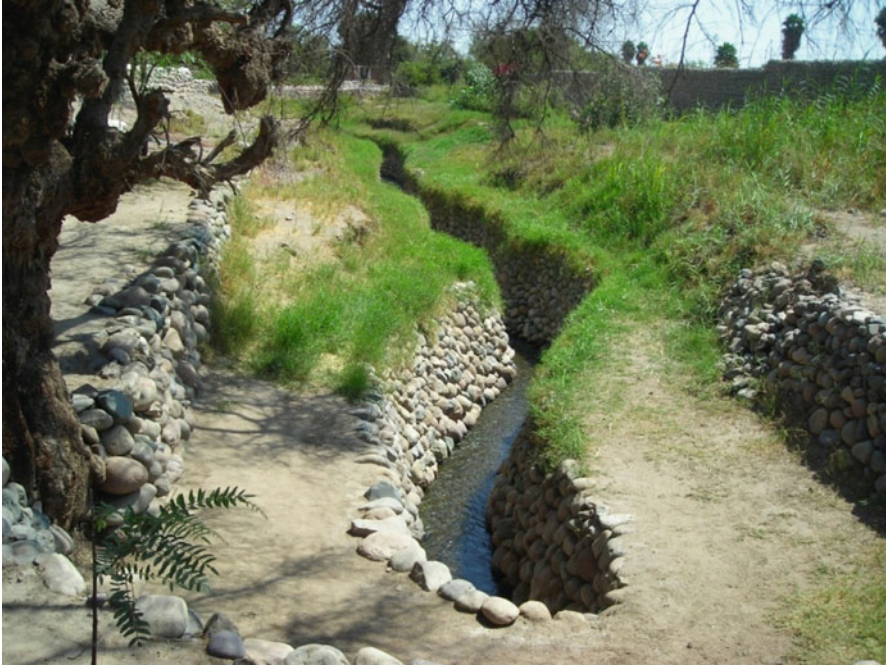
Fig. 12.3 Puquios with the shape of open trenches according to the way the galleries were built
