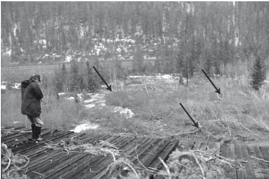
Fig. 2 Tree sampling areas on Shed seven avalanche path ( arrows ). Note downed trees on roof of railroad snowshed man stands on, and on ground beyond snowshed
