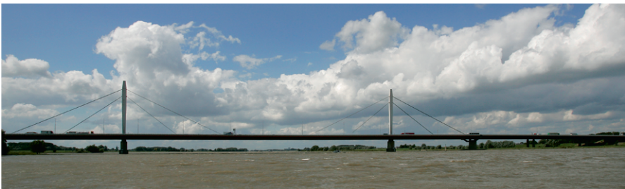
Figure 19.1 Photo of the cable-stayed bridge.
