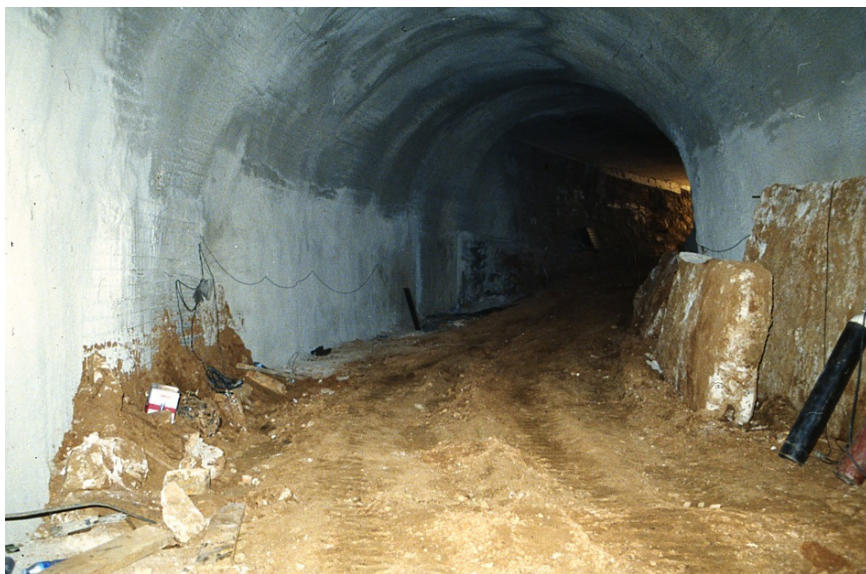
Figure 7.7 The finished tunnel.
